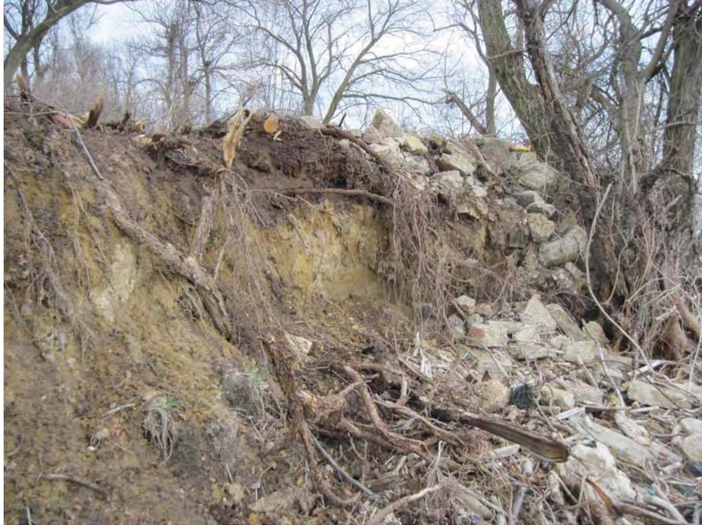
Plate 3. A section of the Army Creek Dike bank eroded from the effects of Hurricane Sandy.
